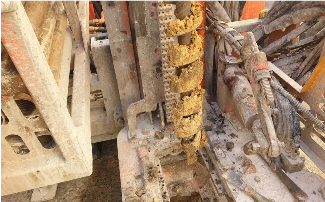
Photograph 5: Representative image of residual clay material encountered within borehole location BH3.M (01.09.20)
